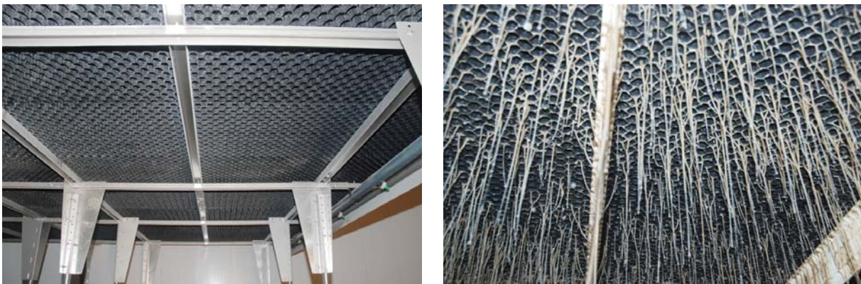
Figure 7-3: Water inflow side clean (left) and excessively contaminated (right)
